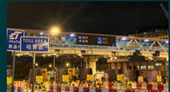
Toll Information Display System (TIDS)
