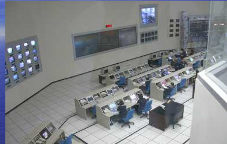
Traffic Control Center - Police
