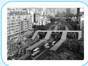
Figure 5-2 | View of BRT Station
